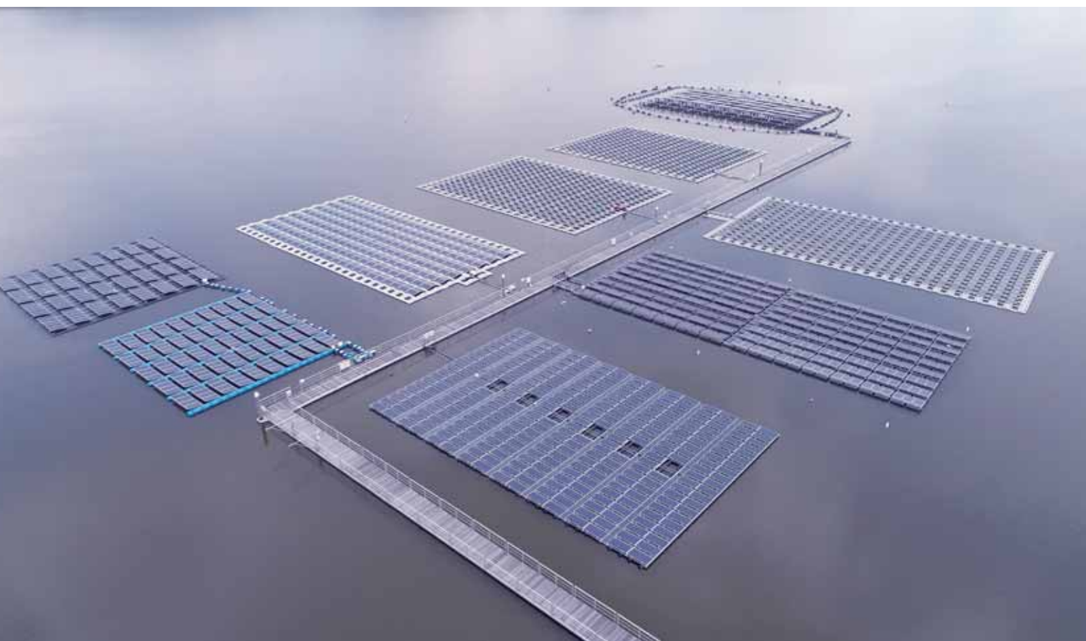
Figure 1. Singapore testbed of 10 different floating solar technologies on Tengoh reservoir
