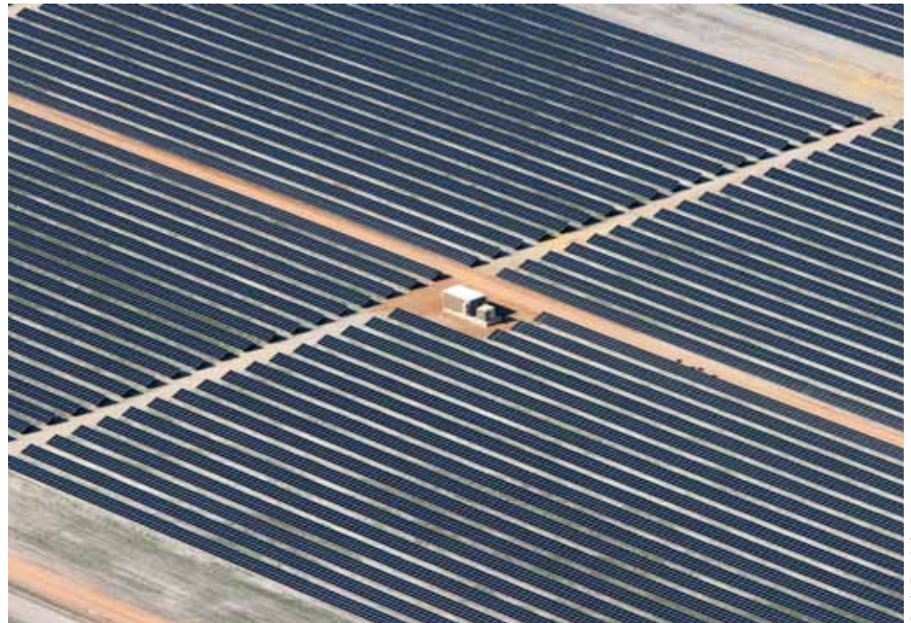
Credit: First Solar
