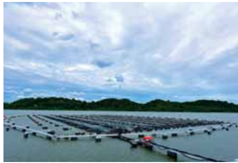
Figure 2. BBR/Solaris testbed system
