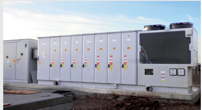
GE's 1500V 'ProSolar' central inverter forms part of the emerging generation of higher-voltage PV equipment.
