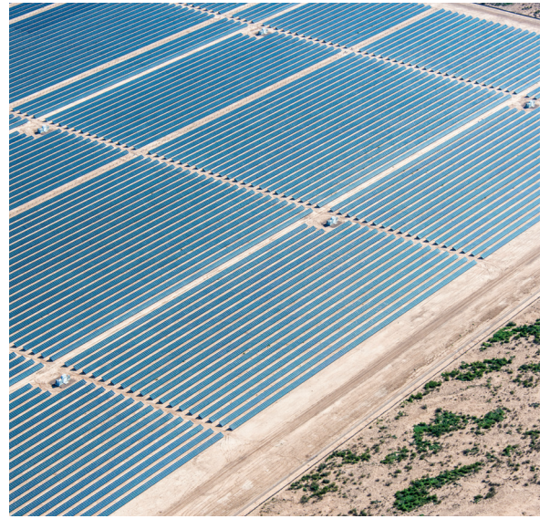
Credit: First Solar
