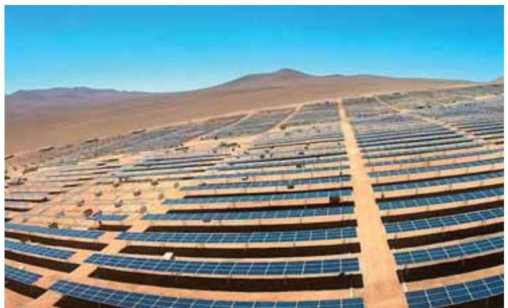
Figure 2. Aerial view of the Lalackama I PV power plant [11].
