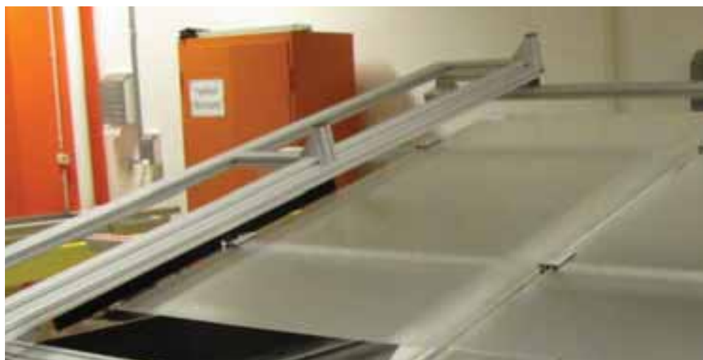
▼ Figure 6. Dry cleaning on the lower glass area.
