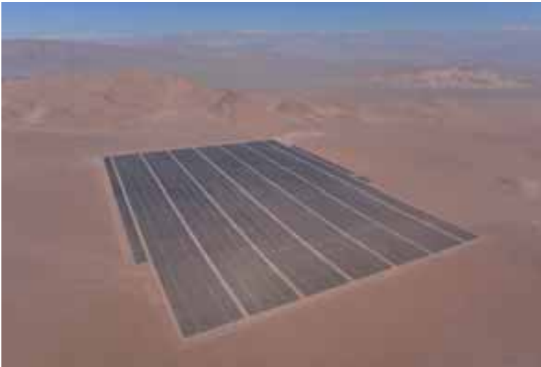
Figure 1. Aerial view of the Amanecer Solar CAP PV power plant [8].
